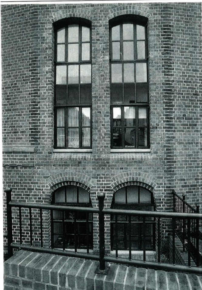
New windows have been carefully matched to the originals.
