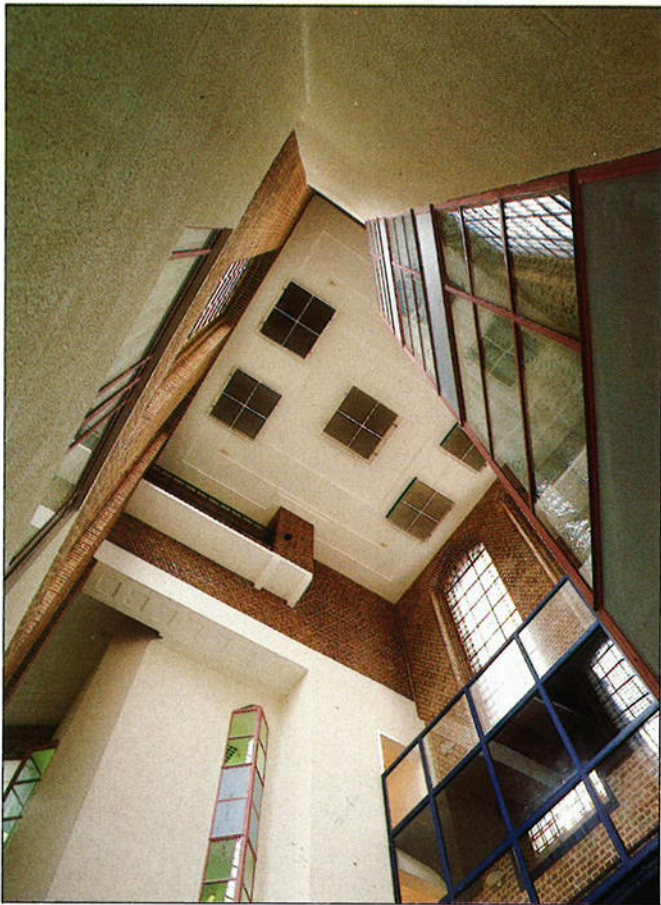
Powerful smoke extractors in the ceiling of the atrium were essential.
